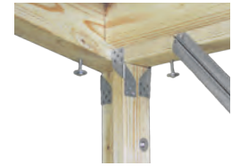
Corner Bolt Connection on Vaulted Wall Building
