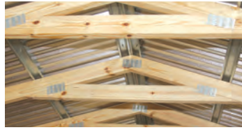
Roof Assembly with Steel Hat Channel
