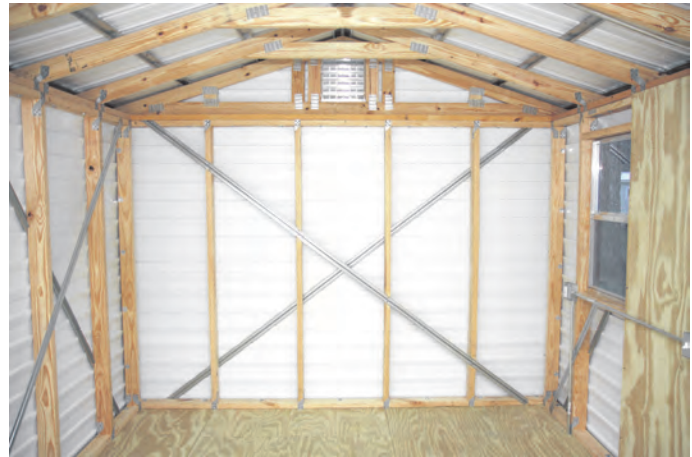
End Wall With Double Top Plate & T Wall Bracing
