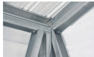
Roof Connection to Side and End Wall
