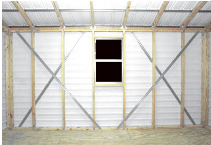
Shear Wall Bracing
