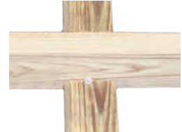
4" Lag Bolt Connecting Crossmember to Skid
