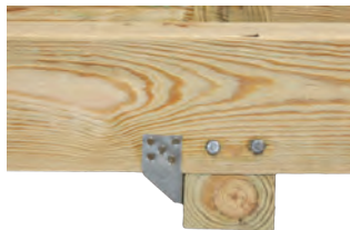
Skid End Double Lag-Bolted and Hurricane Clipped
