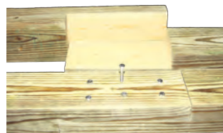
Mortise Splice and Bolted Skid
