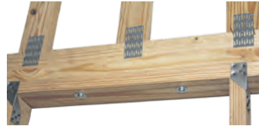
Bolt Connection to Double Top Plate
