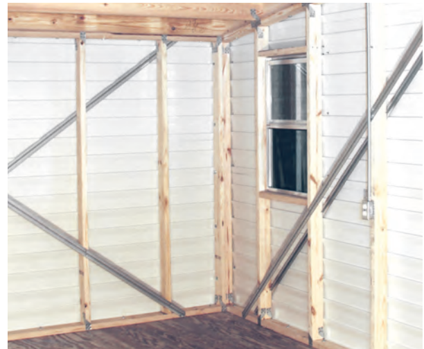
Vaulted Wall & Roof System
