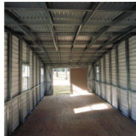
Accusteel Side-Gable Roof and Wall Structure
