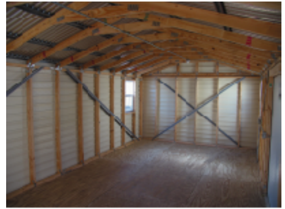
Rectangular Wall Sections with T-Wall Bracing
