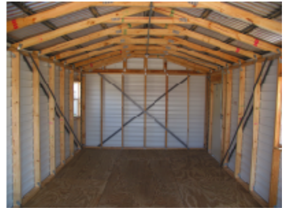
Roof Joist with Collar-Tied Truss Plate Connections
