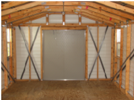
Shear Wall Bracing with 60" End Door
